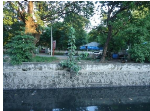
Figure 4 Trash located near Cow Lake Dug Well on the bank of Shwe-Ta-Chaung Creek
